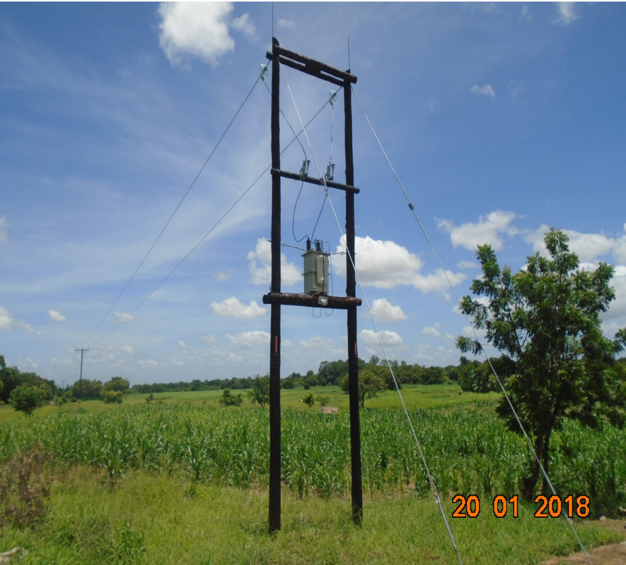
Mini-grid Power lines and a single phase 25KVA step-up transformer at Nyamvuwu
