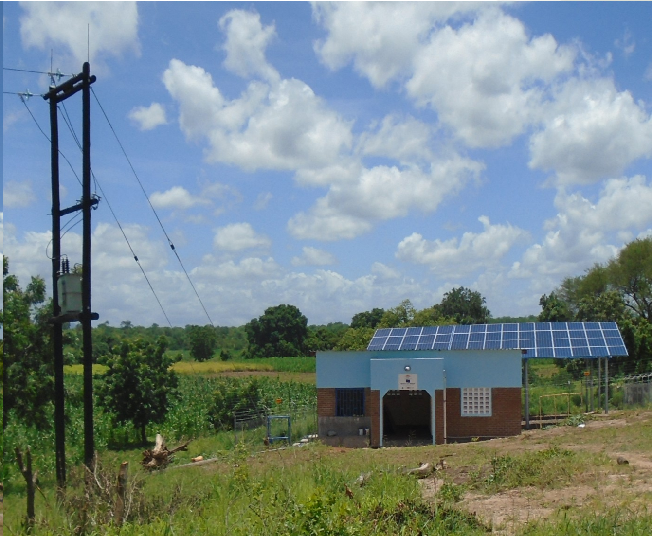
Mini-grid Power lines and a single phase 25KVA step-up transformer at Nyamvuwu
